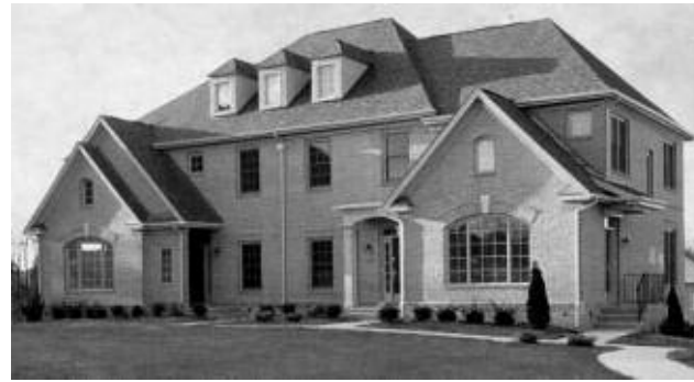
Great House in the Edgemoore at Carrington development in McLean, Virginia
