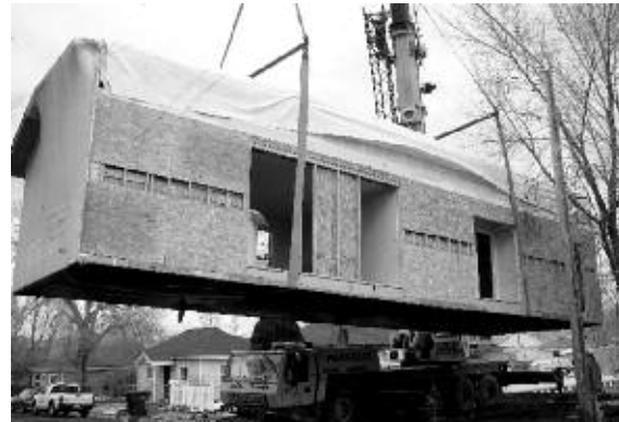
Modular housing being used on infill lots in Magna, UT by Community Development Corporation of Utah.
